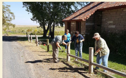
BLM crew constructing fence - by Tim Blount
